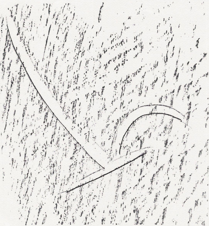
Carpenter's assembly marks
